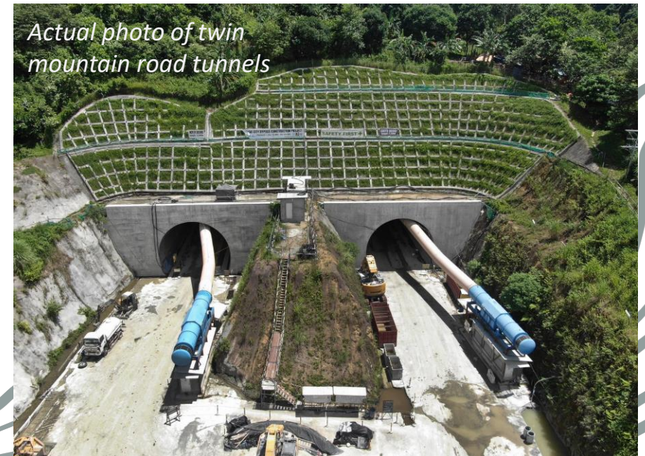
Tunnel Excavation works
