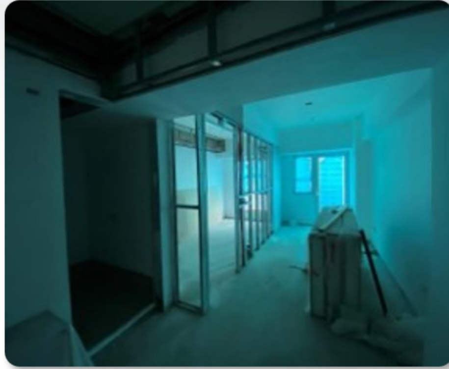
Dry Wall Installation on the 4 th Residential Level in Tower 1
