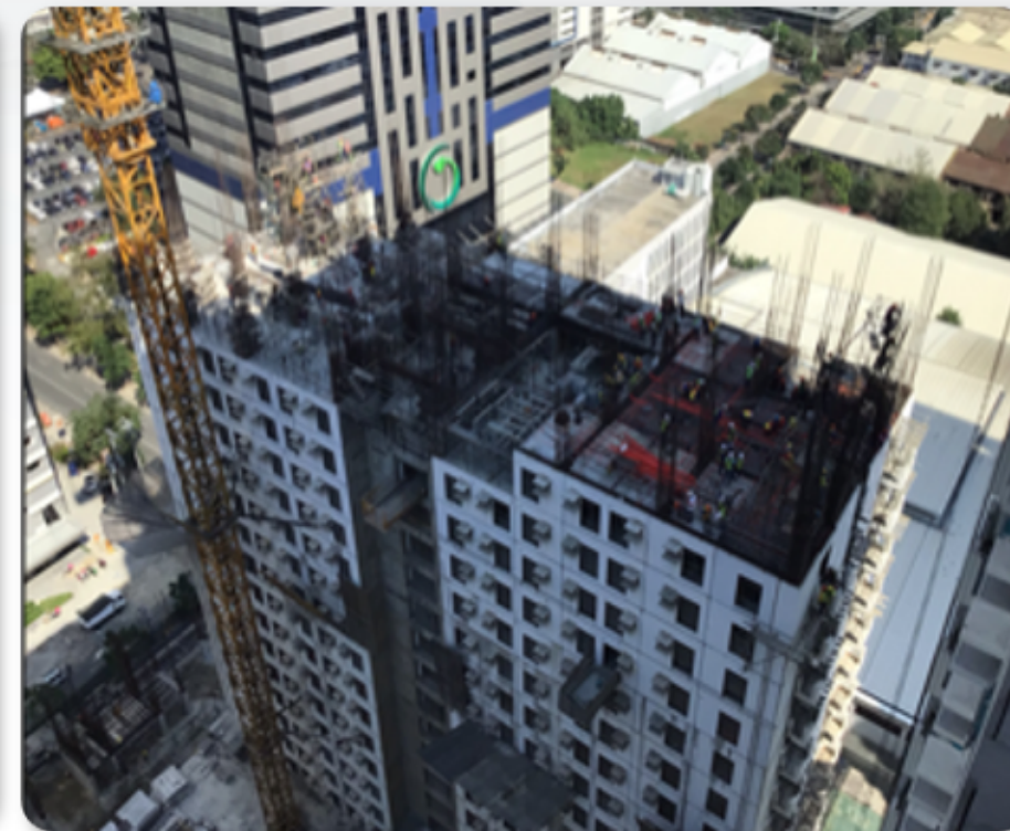
PBU, Rebar Installation and Formworks Installation In Tower 2
